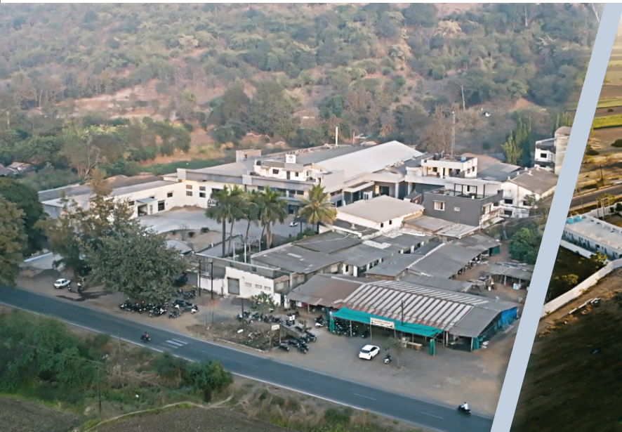
HEX - BCA factory at Vapi, Gujarat
