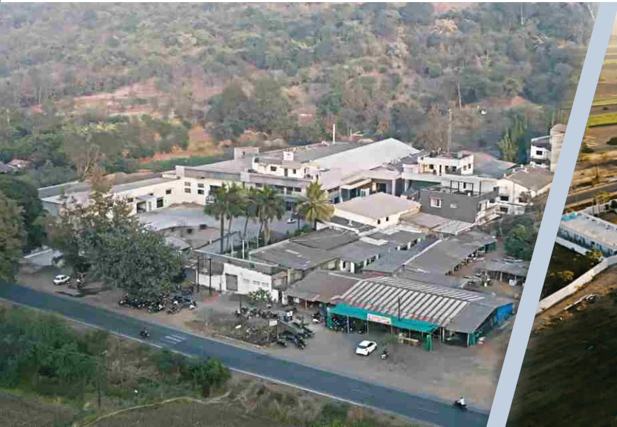
HEX - BCA factory at Vapi, Gujarat
